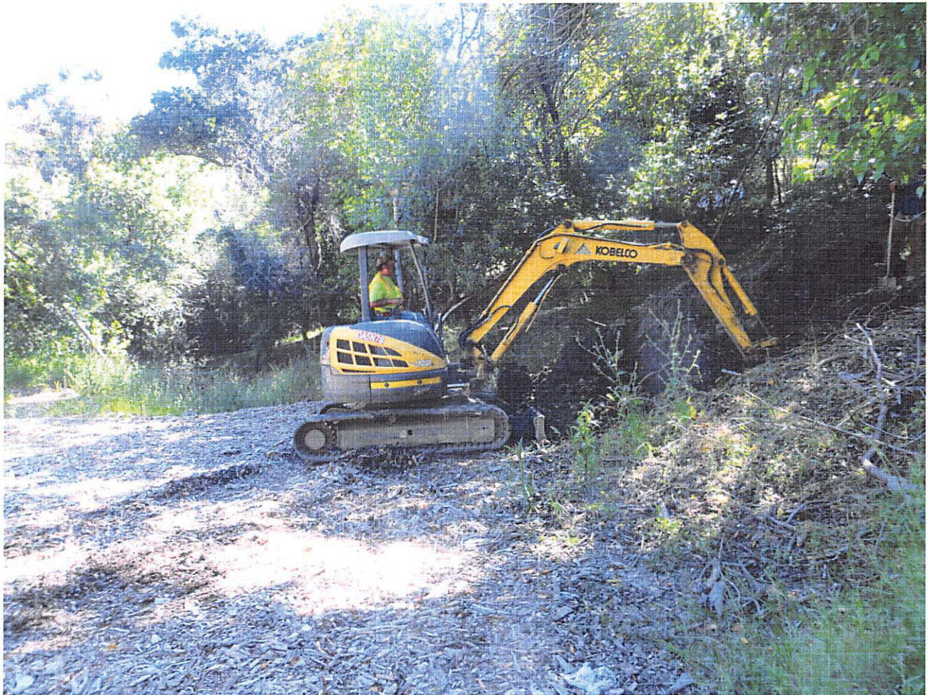
Photo 6: View of backhoe excavating Test Pit 1.
