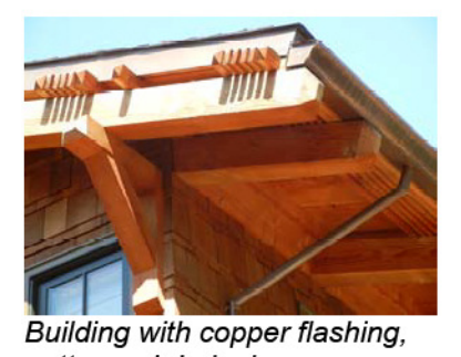
Building with copper flashing, gutter and drainpipe.
