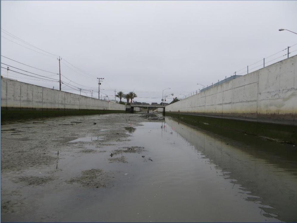
**Photo 5:** Reach 2 looking upstream at the Caltrain railroad bridge. Sediment deposits downstream of the bridge on the left side of the photo, where flow separation and eddying create a depositional environment.
