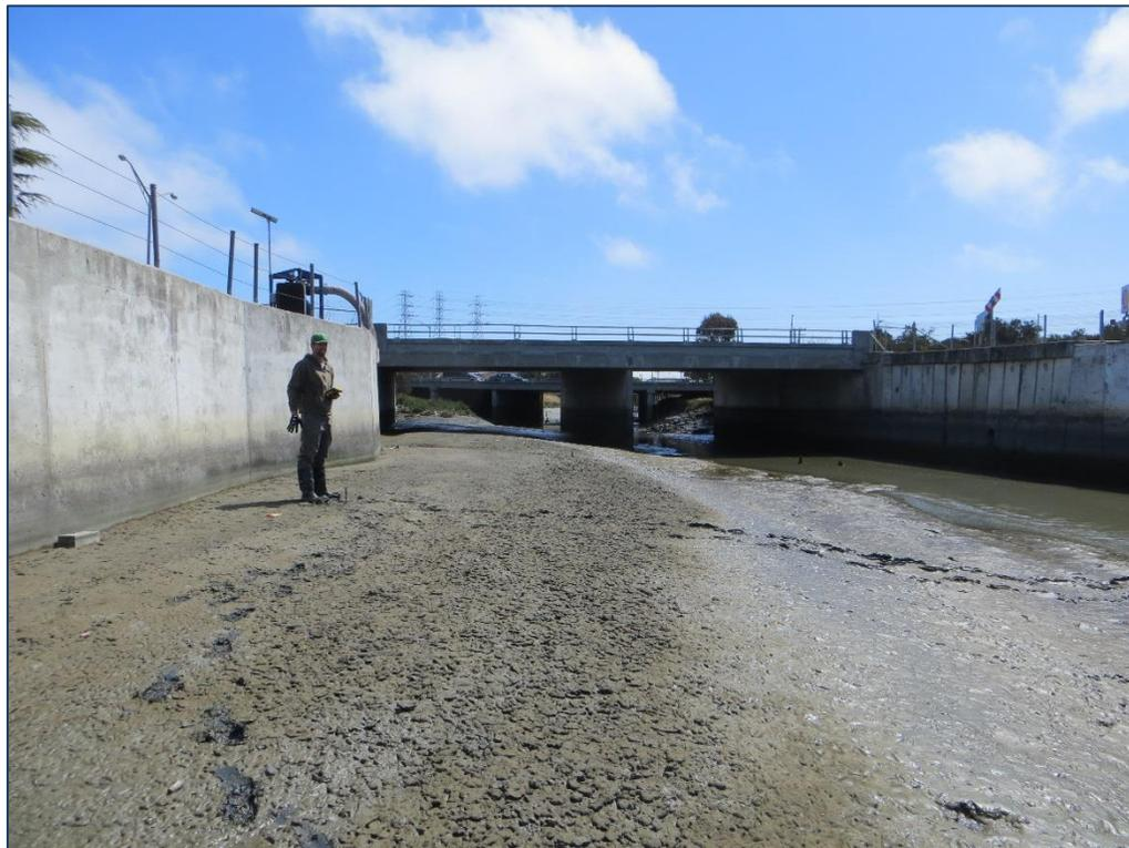
**Photo 7:** Reach 3a looking downstream from Produce Avenue at low tide. Note earthen bed and banks comprised of fine sediment, some depositional bars along channel bed, and mid-bank bench with pickleweed.
