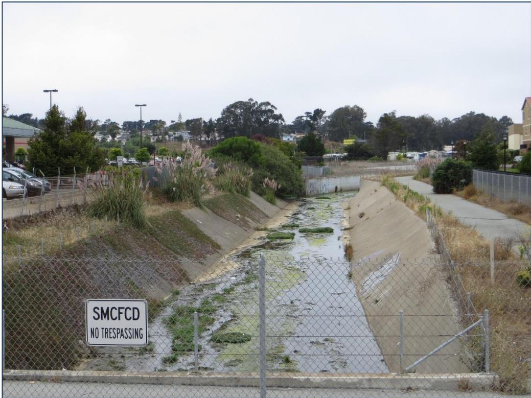
**Photo 3:** Lower Reach 1, at energy dissipater teeth (looking upstream). A small amount of sediment and debris accumulate near the teeth.
