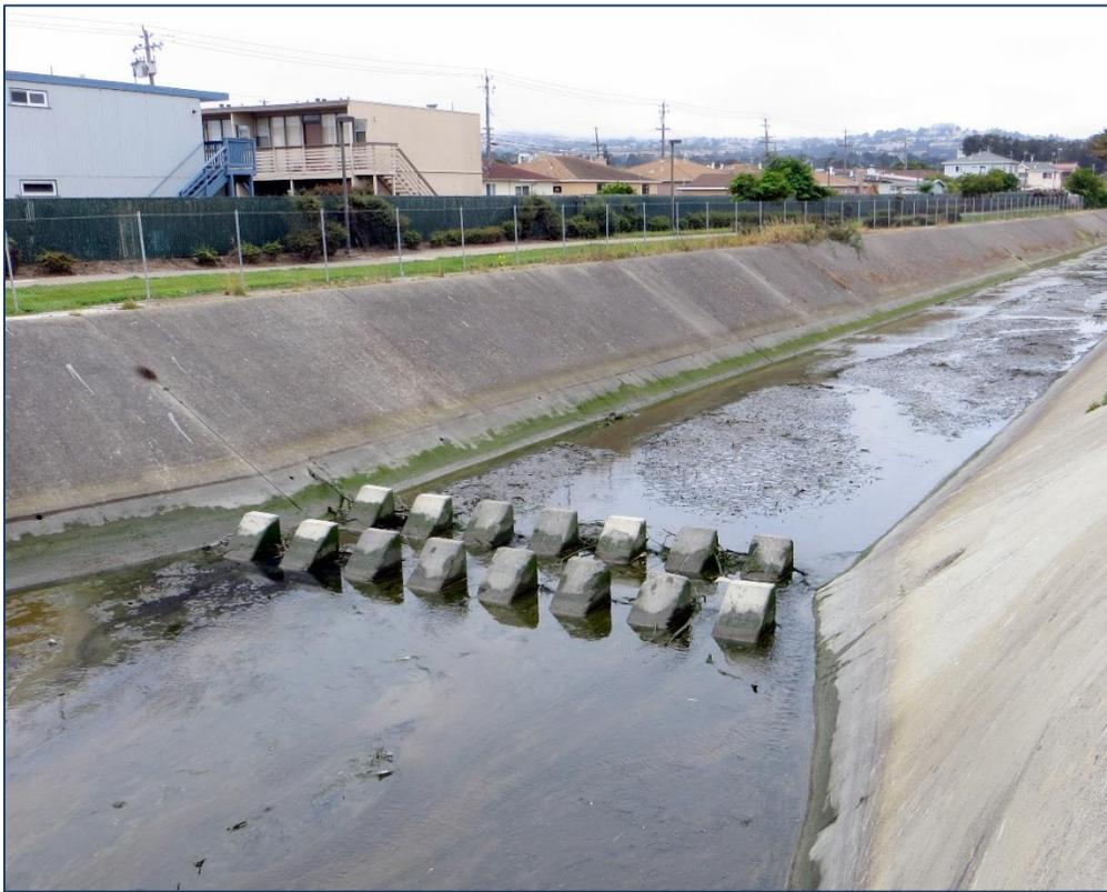
**Photo 4:** Upstream portion of Reach 2 looking downstream near Spruce Ave. Minor sediment accumulation on channel bed.
