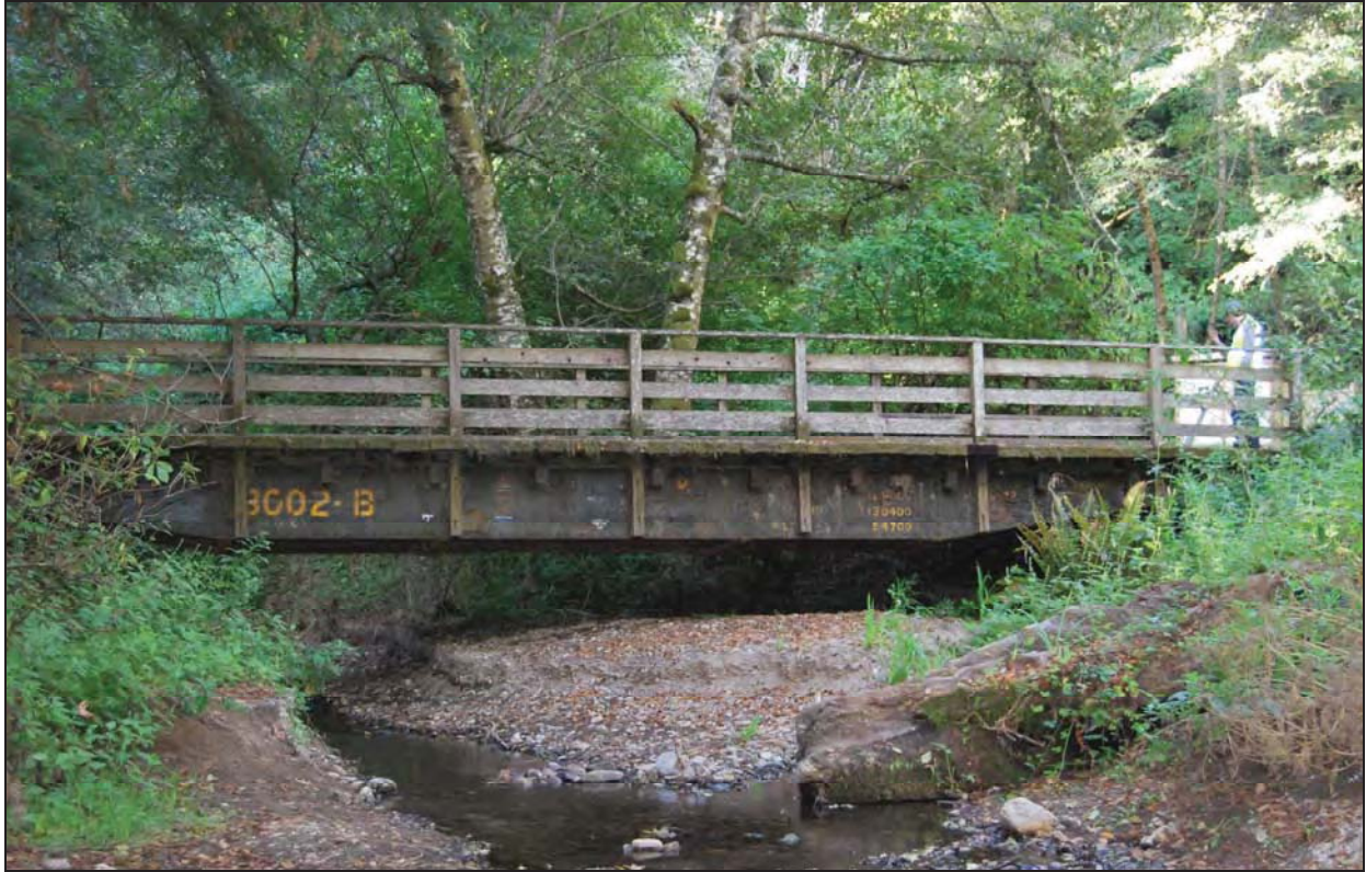
Figure 5: Harkins Bridge, view east
