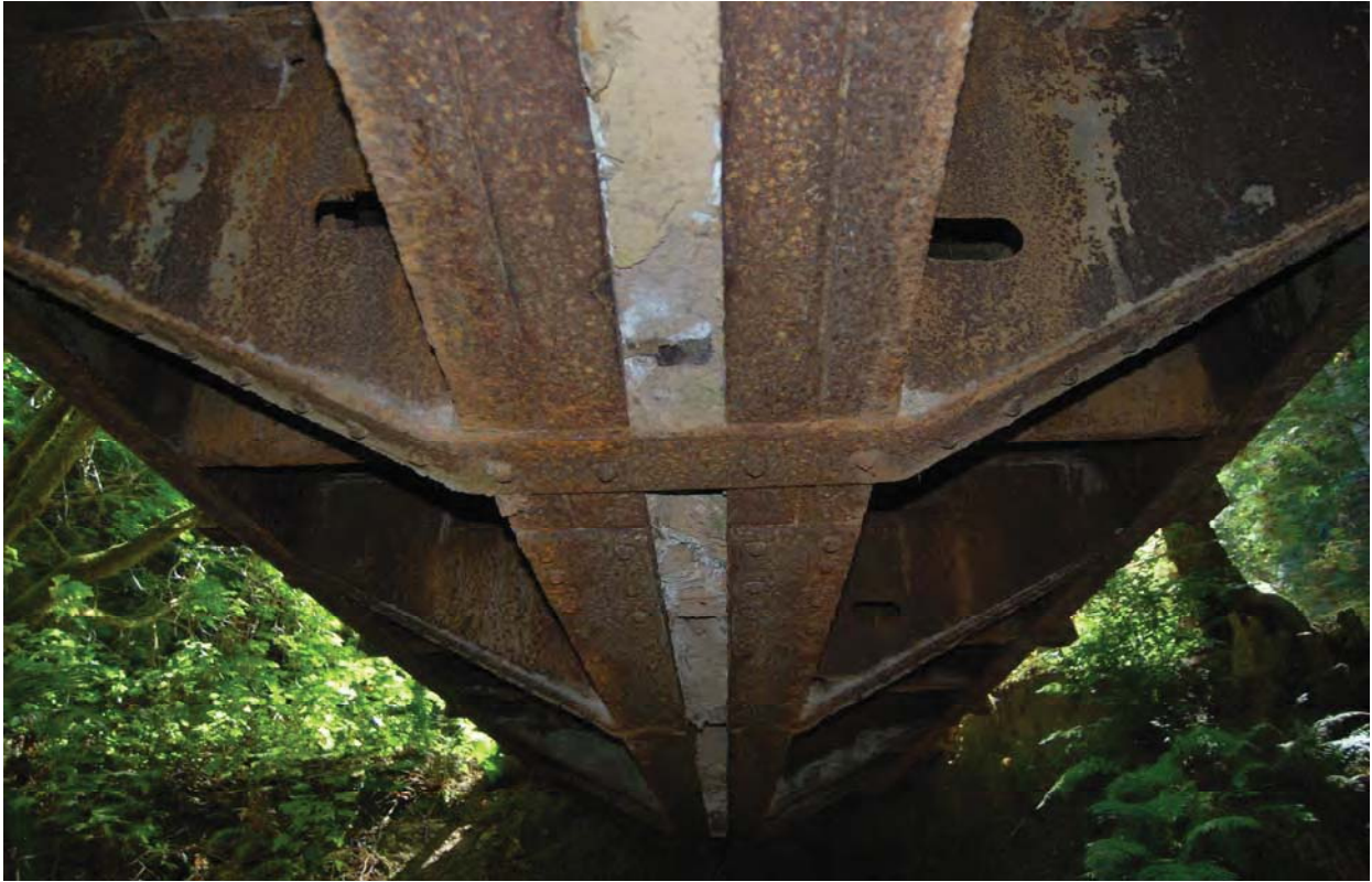
Figure 9: Purisima Bridge 1, view of redundant main box girder and stringers
