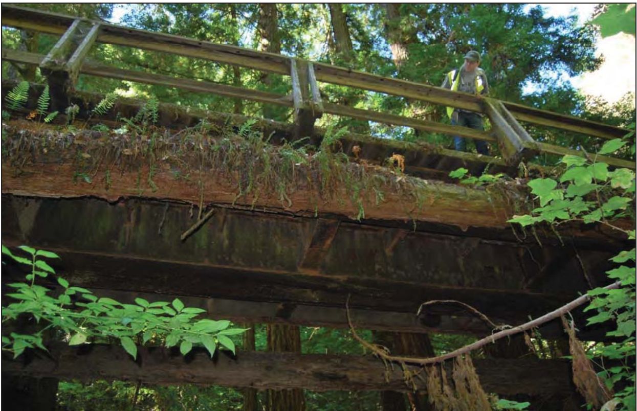
Figure 12: Soda Gulch Bridge, view north and below
