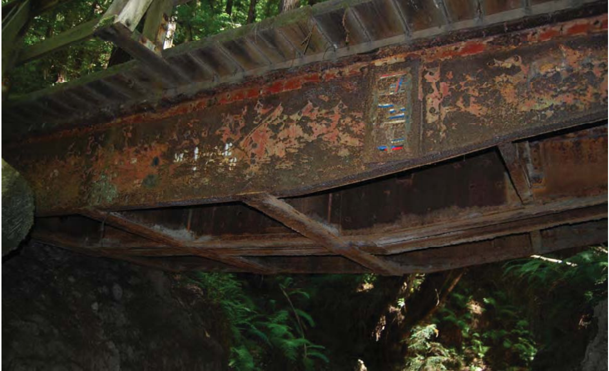
Figure 17: Purisima Bridge 2, view of exterior girders, stringers, and main box girder
