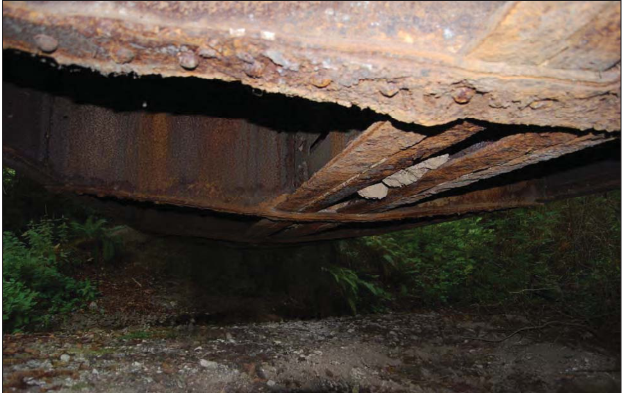
Figure 6: Harkins Bridge, redundant box girder and stringers
