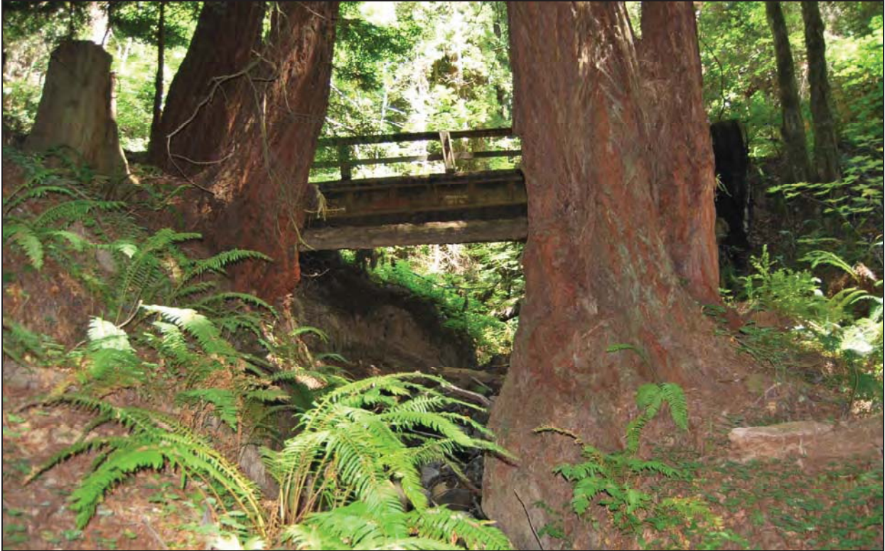
Figure 11: Soda Gulch Bridge, view north
