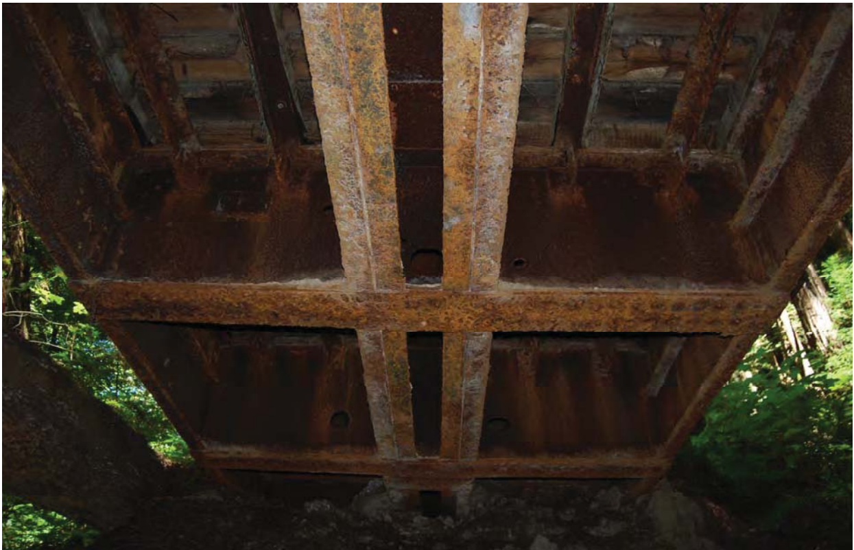
Figure 16: Purisima Bridge 2, redundant main box girder and stringers
