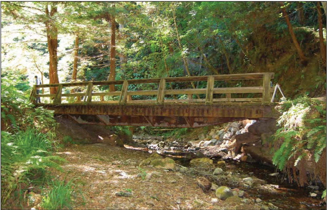
Figure 8: Purisima Bridge 1, view south
