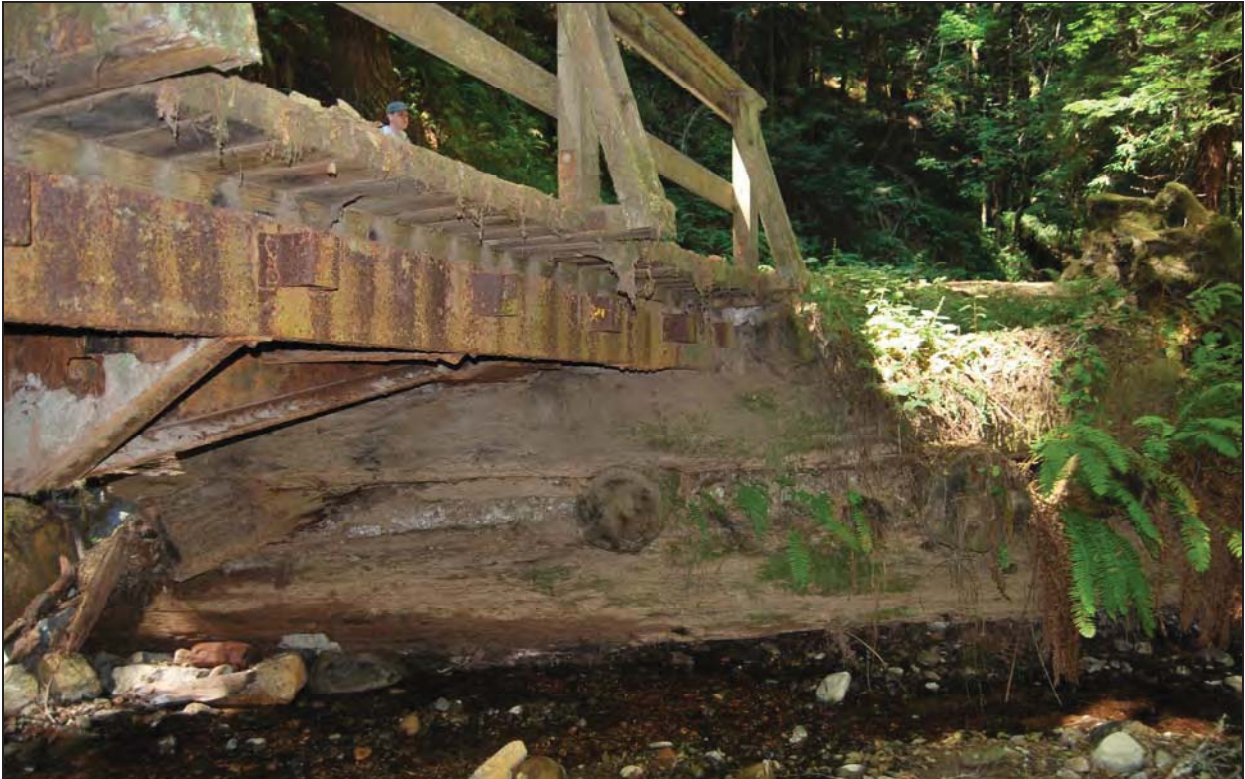
Figure 10: Purisima Bridge 1, view west at redwood abutment
