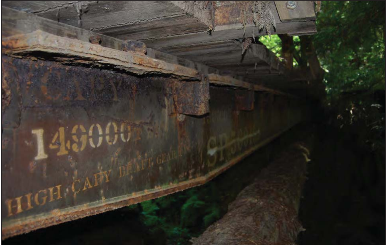
Figure 14: Soda Gulch Bridge, exterior girder with markings (SP 509193)
