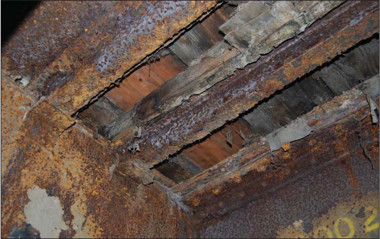
Figure 7: Harkins Bridge floor beams, exterior girder with markings (SP 13002-B)
