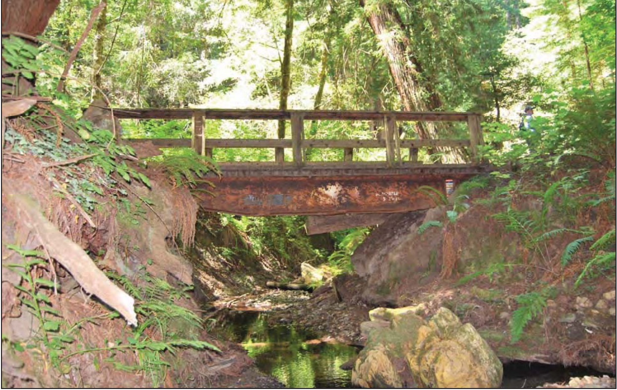
Figure 15: Purisima Bridge 2, view south
