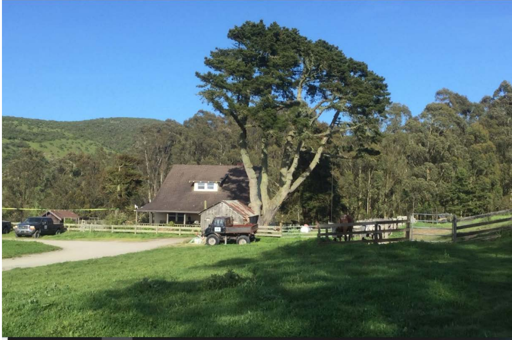
Location C-Existing single family house
